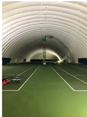
Installing the insulation
